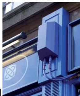
Microcell providing extra capacity in town centre
